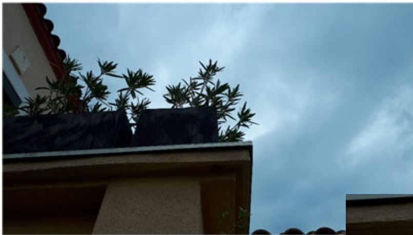
Figure 3-1 under exposure useless for inspection
