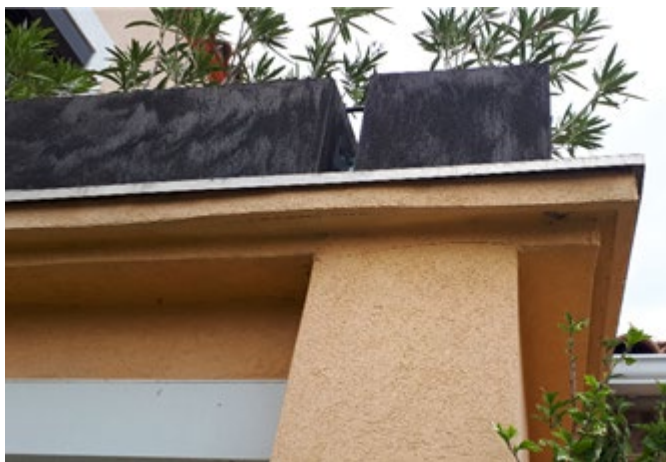
Figure 3-2 good exposure for the inspected area
