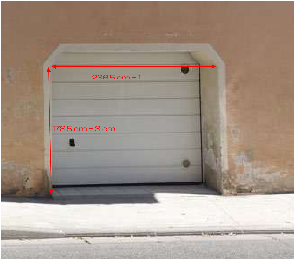
Figure 5-21 dimensions measured on a door
