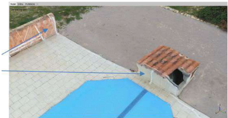
Figure 6-12 tiled model defaults on the pool's wire fence
