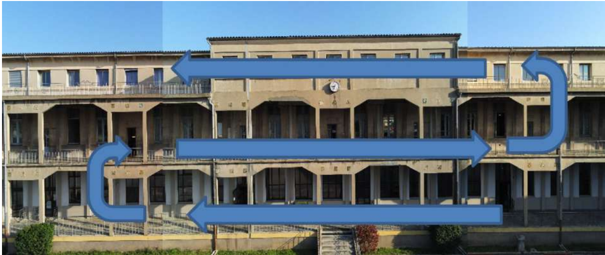
Figure 3-10 path for façade photogrammetry
