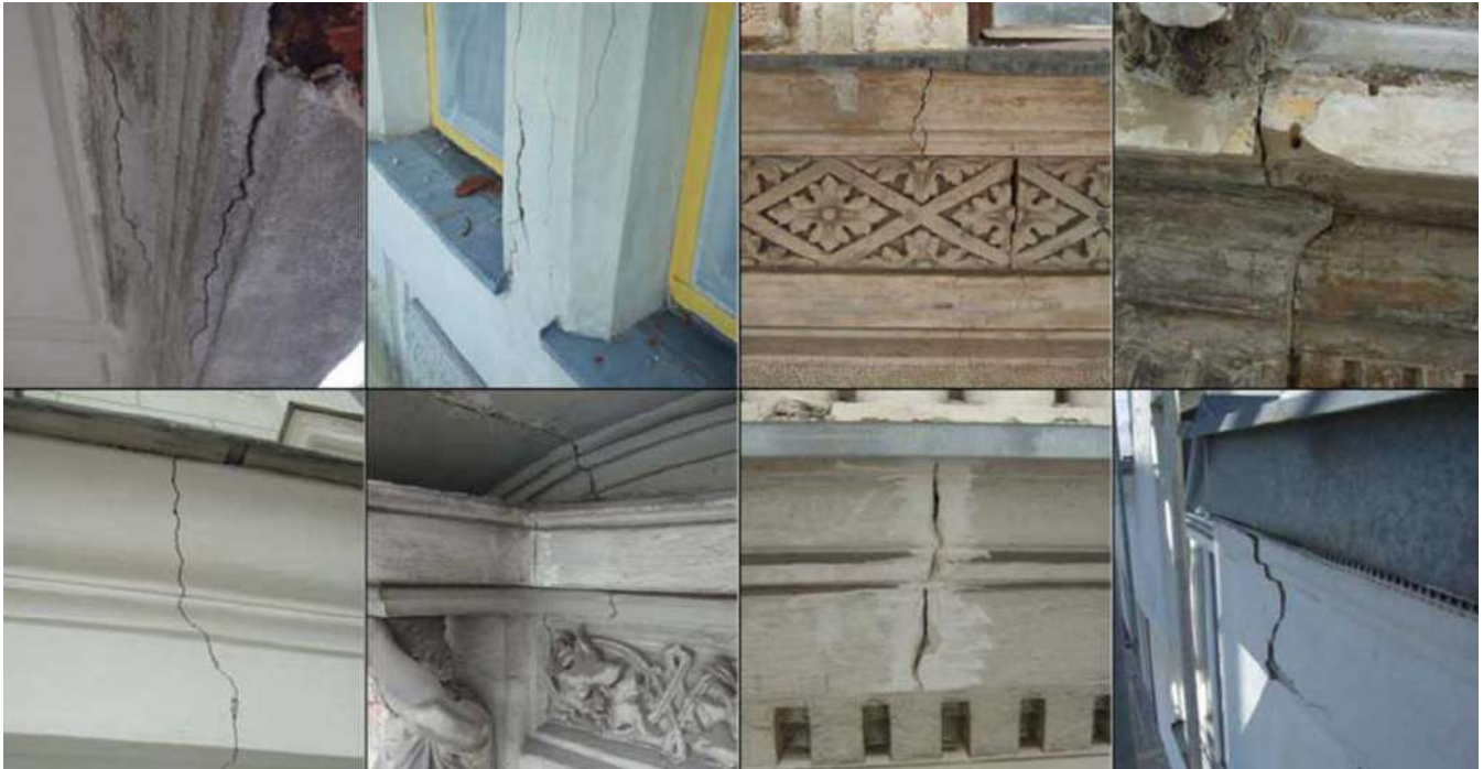
Figure 2 Typical damages on facades ( https://www.zukunft-bau.at/bauschadensberichte )
